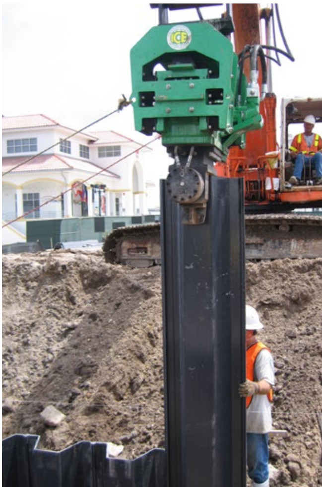
Vibratory Hammer Installation Example
