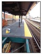
The decking was manufactured with an integrated tactile warning strip and an ADA compliant antiskid. The decking panels were pre-assembled into 48" wide modules and sent to New York City where they were installed in March of 2012.
