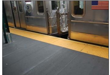
New York City Mass Transit Authority Engineers recognized the need to repair and replace the 45th Road, Courthouse Square elevated rail platform with a lightweight limited maintenance decking system. The decking system was required to replace the existing deteriorated concrete deck, which was spalling and crumbling, resulting in debris falling fifty plus feet onto vehicles and sidewalks.
